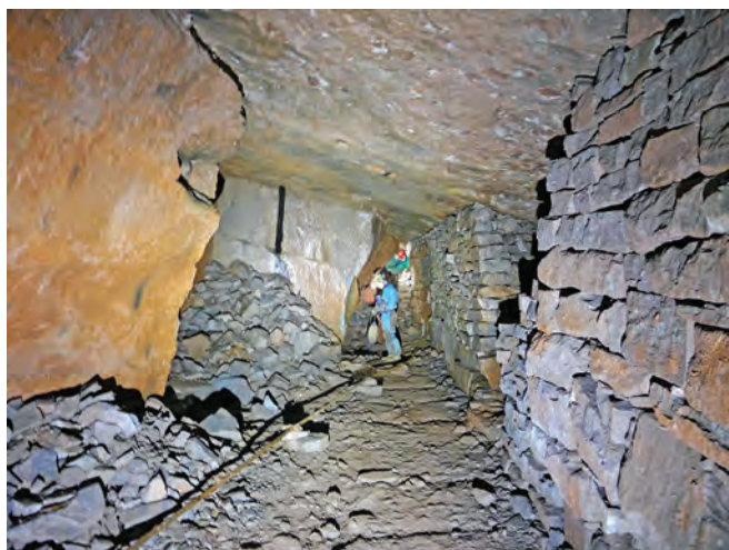
Blakeney Hill: SubBritters negotiating the Cold Draught Wall in Old Upper Level, viewed from Split Stone Chamber At the far end of Old Upper Level, along which sleeper impressions were still evident, we descended, skirting the Old Mid Workings where the roof is in a parlous state, to reach the Lower Level with its high walls of neatly stacked deads and a number of tall timber roof props, some with chains attached.
